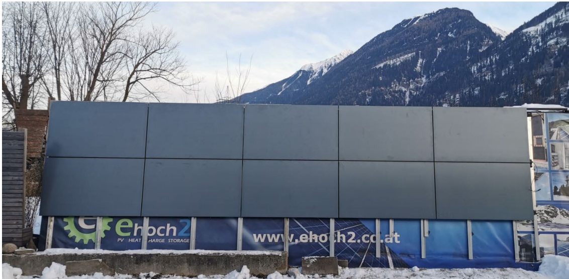
Photo of the test façade with grey screen-printed modules.
