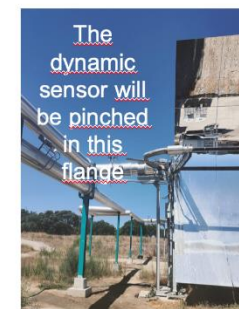
Online corrosion monitoring system onto the molten salt tank
